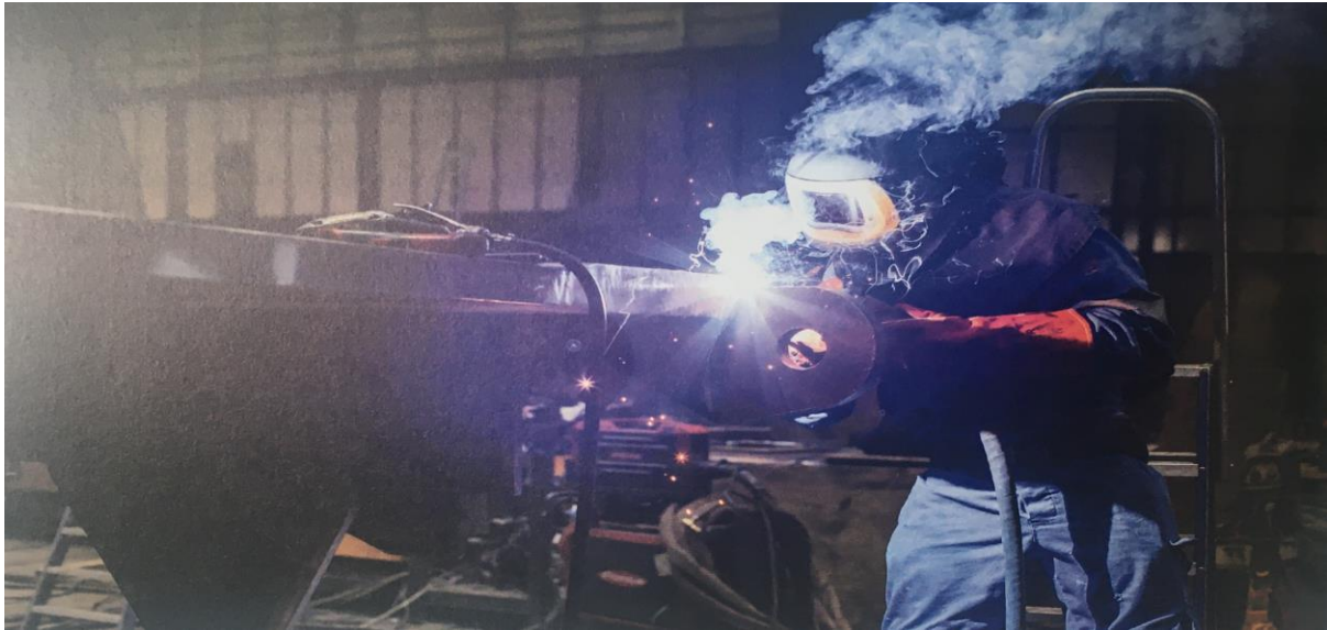
Welder constructing lifting lug in crane for crane-foundation
